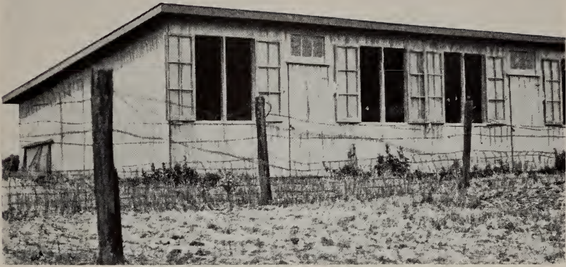
Fig. 15. Glass window sash offers best protection against winter storms and winds. These lie flat against the house front when open, admitting maximum sun.
